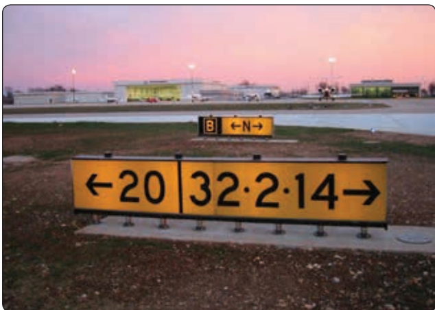
Figure 14-23. Runway destination sign with different taxi routes.
